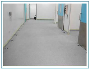
Stonshield HRI mortar base installed with undercoat and broadcast prior to application of sealer coat for final finish
