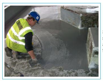
Stonchem 500 Series Topcoat spread out with notched trowel and then back rolled with roller to remove lines.
