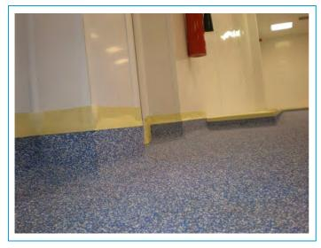
Stonclad GS mortar is used to form the cove profiles allowing a seamless transition and to facilate cleaning. Vinyl Flakes are then applied onto the coves.
