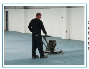
Stonclad mortar applied using a screed box and power trowelled to give a very compact mortar with an even finish and a short installation time.
